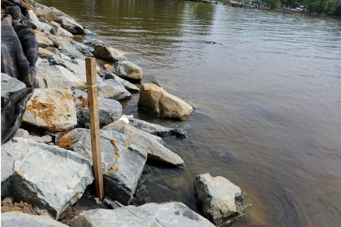
Figure 3 Rip rap stone observed beyond installed stone revetment
