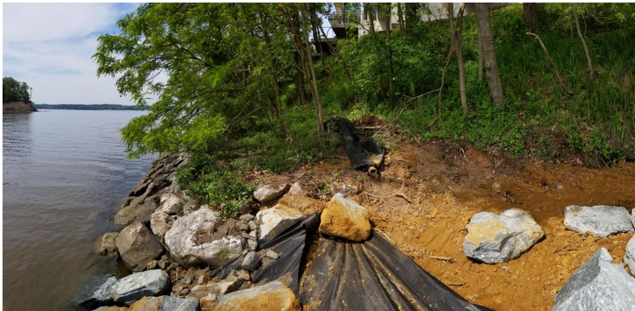
Figure 2 Panoramic view of the existing revetment connecting to the to be constructed revetment (facing S perimeter)
